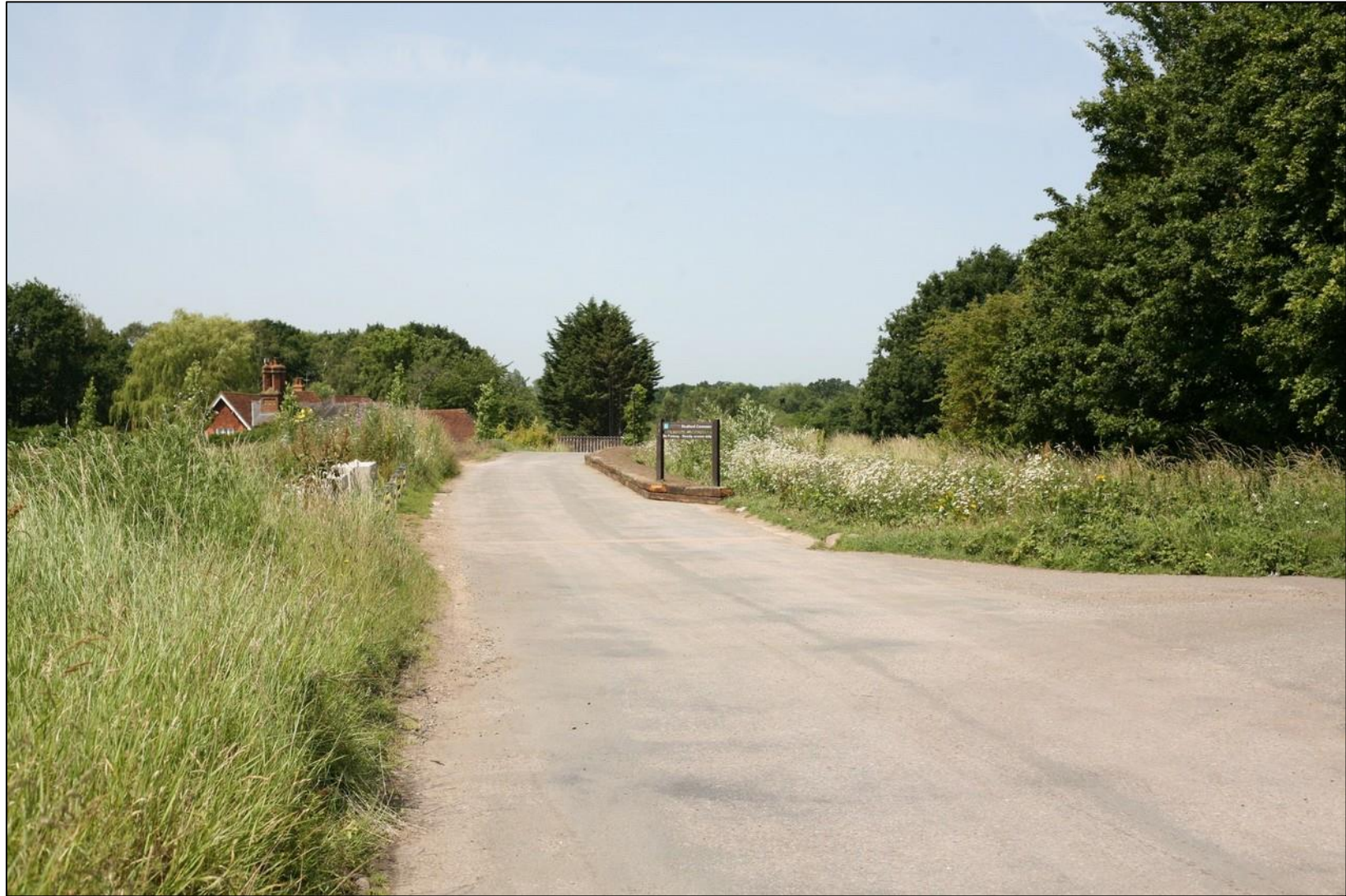
Dagley Lane looking from Horsham Road
